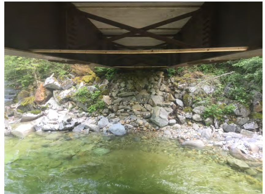
Left Bank Abutment when facing downstream
