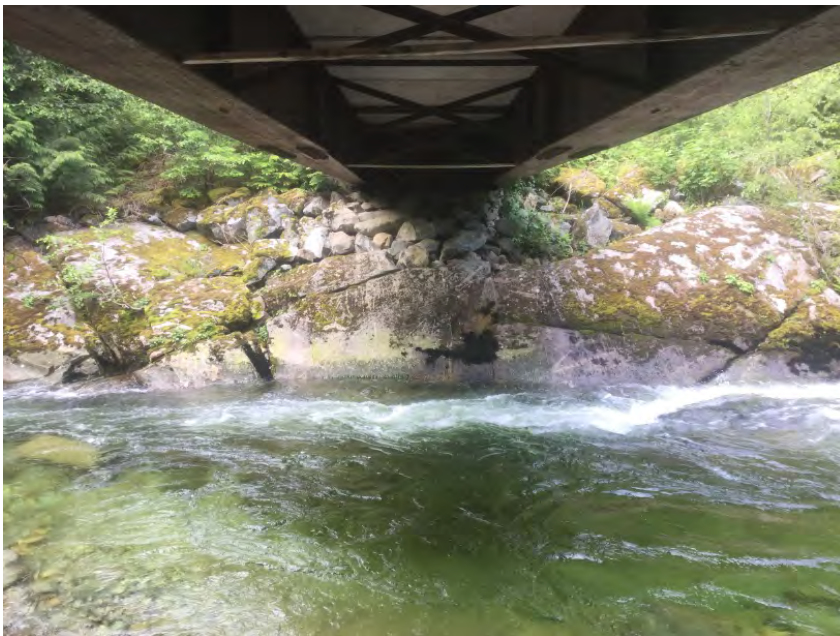
Right Bank Abutment when facing downstream
